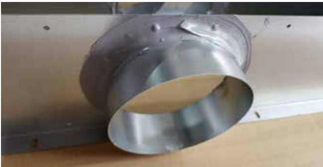
Images: Sealing of joints and flange connections in air ducts.
